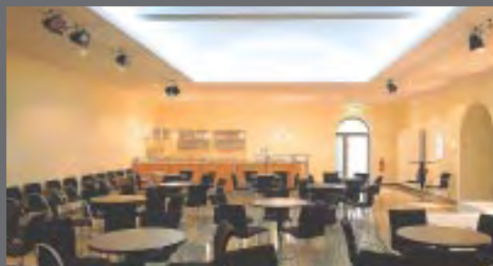
Fiberstars simulates the northern sky in the VIP lounge at the State Theater in Braunschweig, Germany
