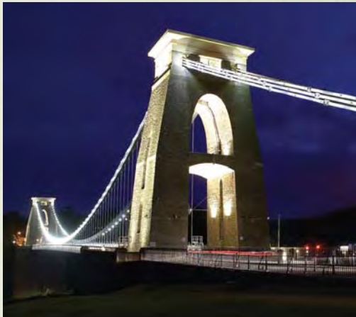
Right - Fiberstars Crescent LEDs on the chains of the Clifton Suspension Bridge in England won an award for lighting designers Pinniger and Partners.
